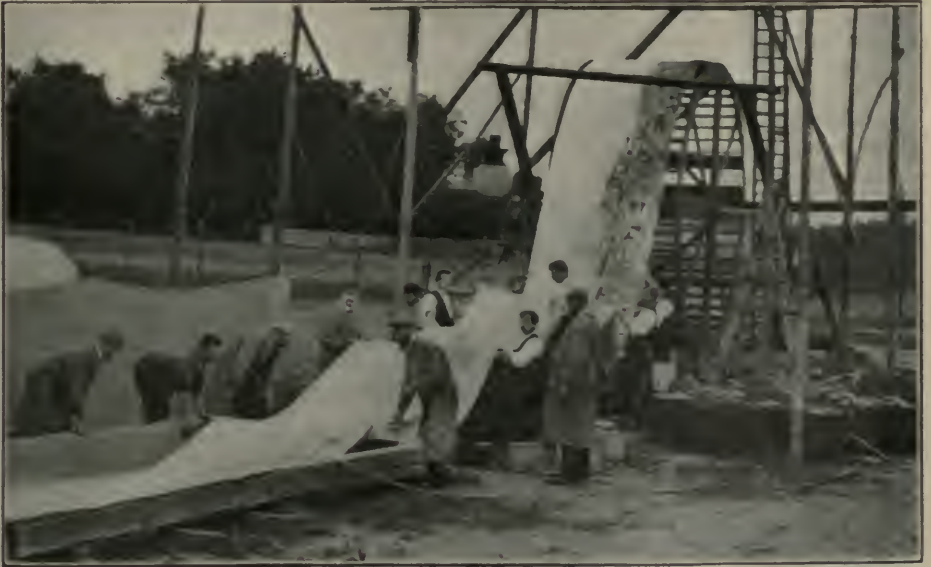
HOW THE LARGEST PHOTOGRAPH IN THE WORLD WAS DEVELOPED The wheel built for the purpose had a periphery of forty-one feet
